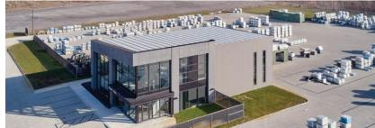
The focal point of Techo-Bloc is its stunning glass and aluminum curtain wall that serves as the centerpiece of the design. Exposed steel beams are becoming increasingly popular in modern designs, and this structure embodies that contemporary vision perfectly. Nucor Building Systems provided three flat beams to create a 4' projection canopy at the striking façade. The canopy has a 9' clear height and is roughly 1' in-depth and thickness.
